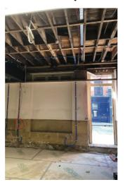
was taken. This revealed nearly 18 inches of extra head room once various services were accommodated. The opportunity to enhance the ventilation system, to bring the electrical and fire detection systems into compliance with current health and safety requirements and to install state of the art lighting with audio visual capability was greatly welcomed.
